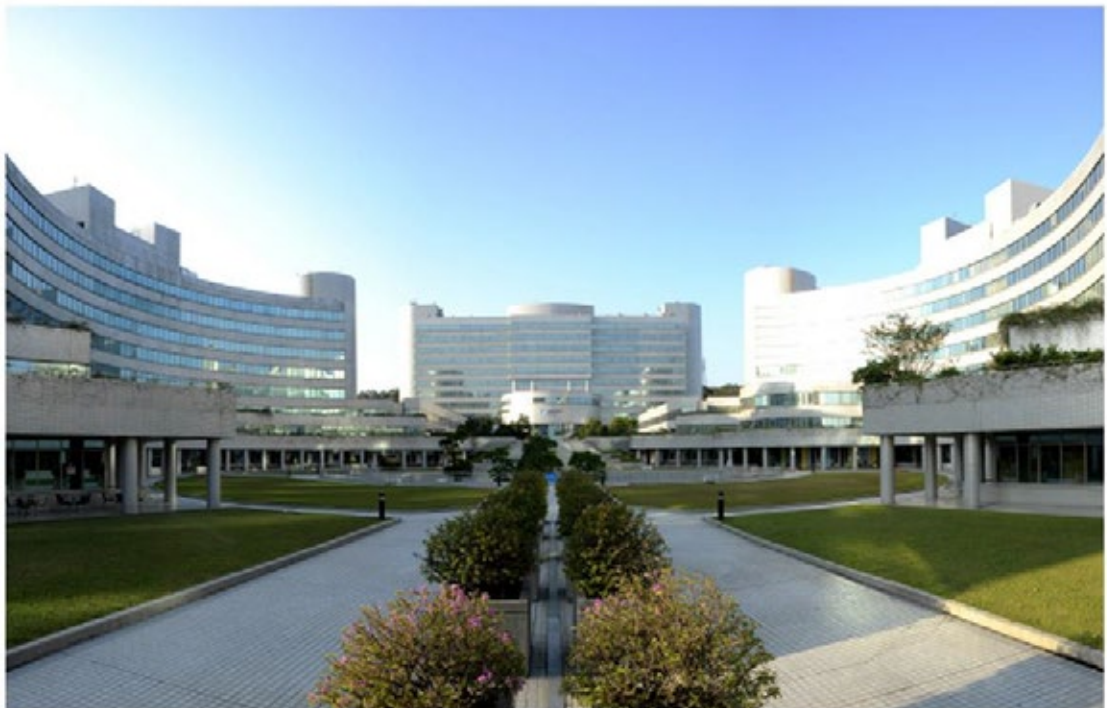
ITRI Main Buildings
